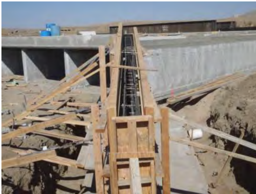
Figure 2-3: Bena Bridges During Construction
