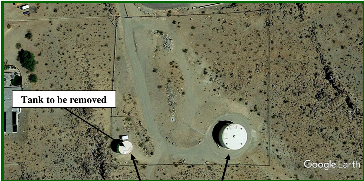
Enlarged aerial view from approximately 2,700 feet altitude (Image date: 7/1/2017)
